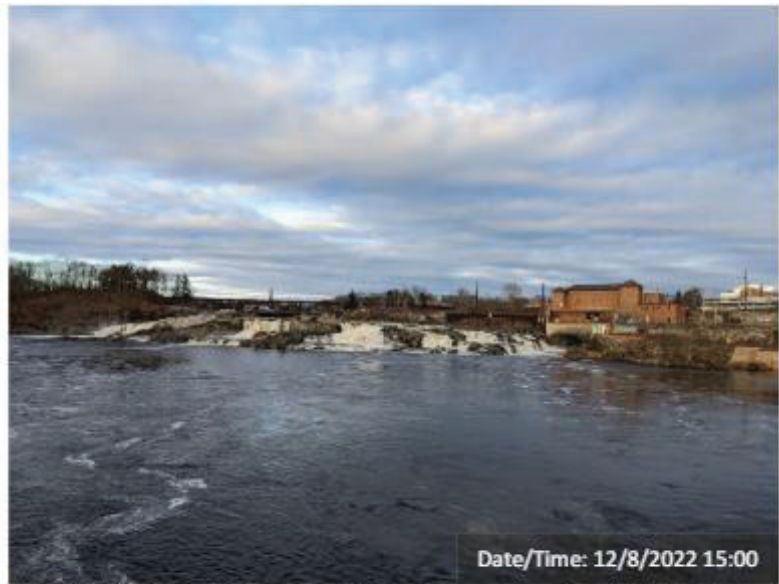
4,350 cfs spill, Dam 1 deflated, Headpond el. 168.29 ft
